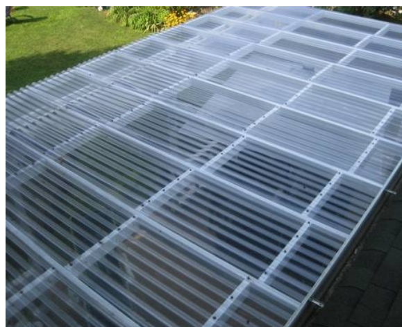
Roof over patio.
