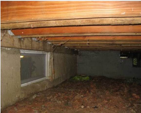
View under the deck. Looked ok.
