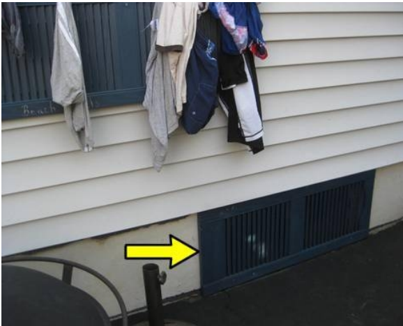
Sealed access to crawlspace.
