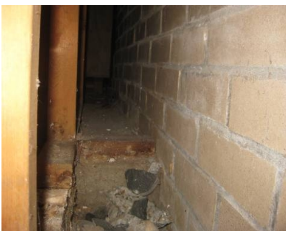
wall behind washing machine wall.
